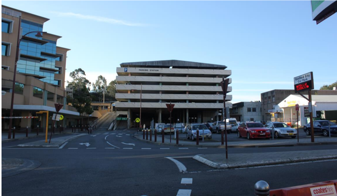
Figure 14: View of Baker Street from intersection of Donnison Street looking north
